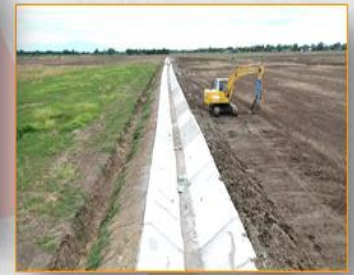
CONSTRUCTION OF TRAPEZOIDAL & RECTANGULAR CONCRETE CANAL LINING & APPURTENANT STRUCTURES (STA. 0+000-STA. 1+203.80) OF LARIS-SUB LATERAL B-2 A
