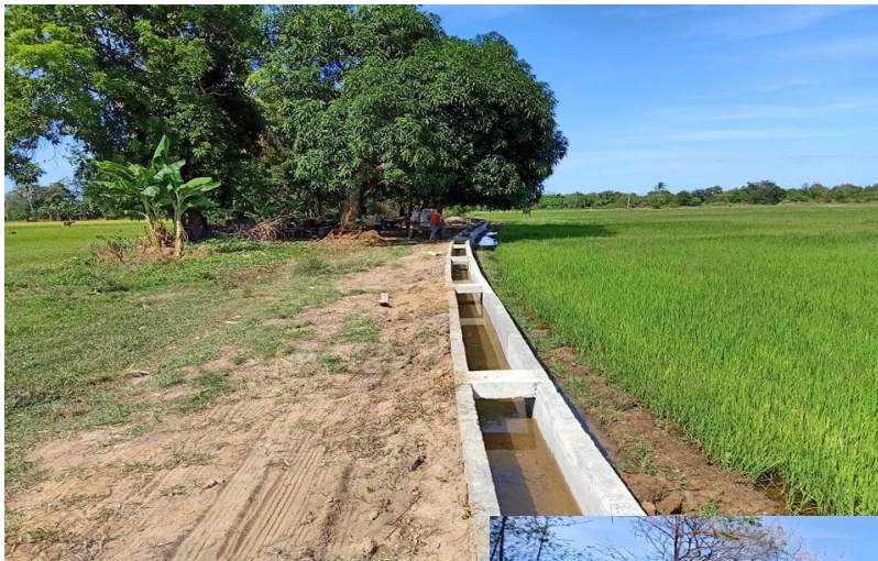
Completed Benchflume CABANO SRIP
