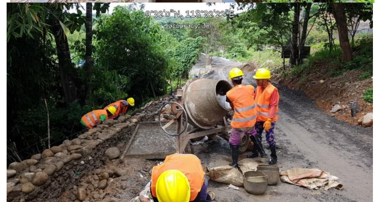
Access Road with Slope Protection
