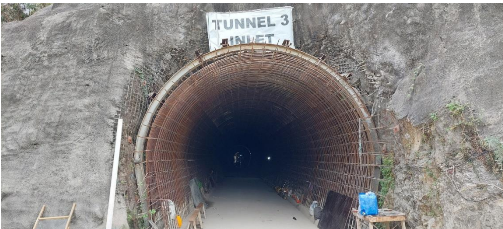
Ongoing construction of Tunnel 3
