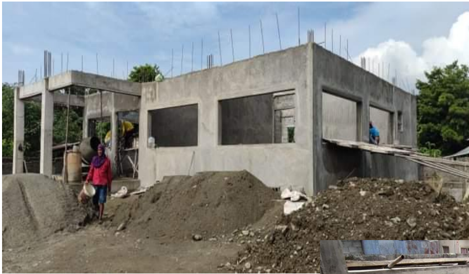
Construction of Field Office, DUMULOC SRIP
