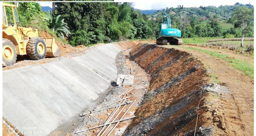
Ongoing Construction of canal lining
