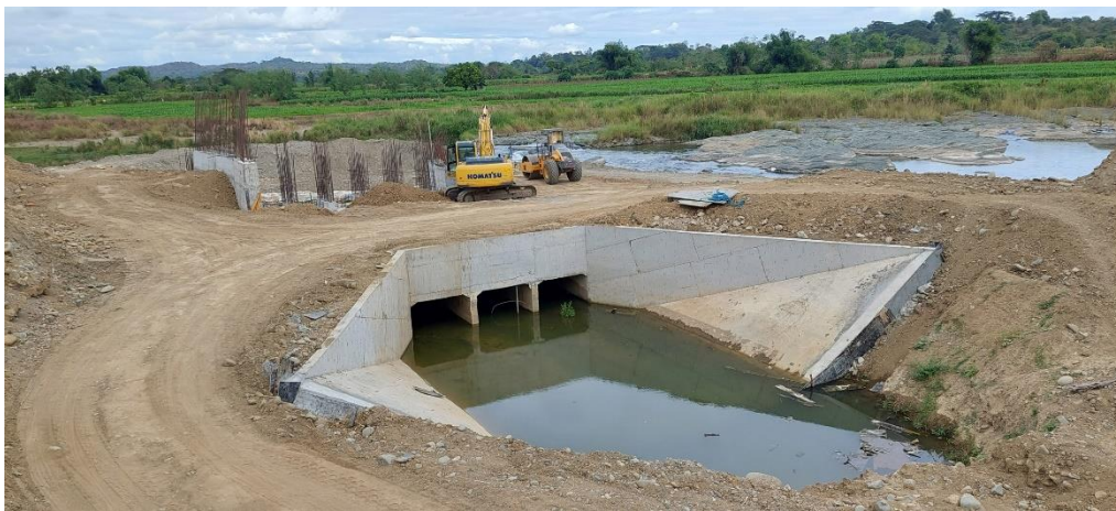
Ongoing South Main Canal
