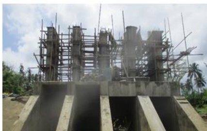
ON-GOING REHABILITATION OF DAM
