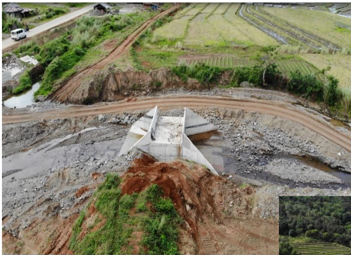
Construction of Drainage Structures & Embankment Compaction @ Main Canal
