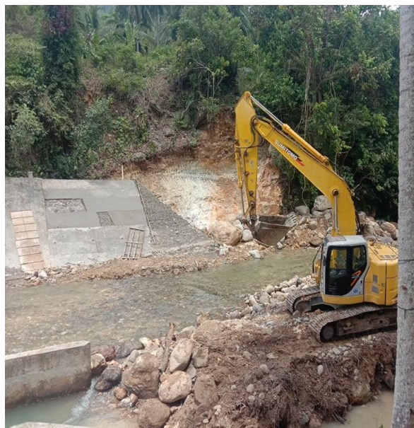
Slope Protection works and canalization works
