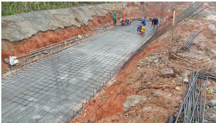
Ongoing Construction of floor slab of closed conduit
