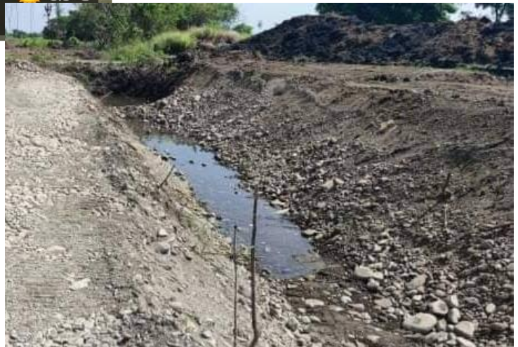
Construction of Canals BAYAOAS SRIP
