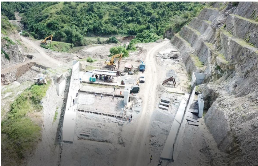
Spillway structure, BONOT-BONOT SRIP
