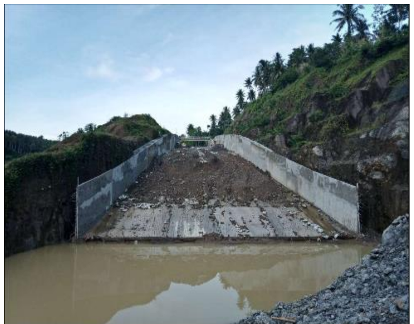
Gravel Bedding & Riprap, Spillway Area IBINGAN SRIP
