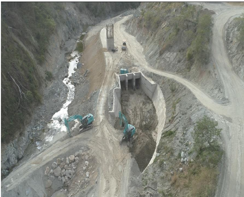
Ongoing construction @ Spillway Area & Diversion Conduit, SULVEC SRIP
