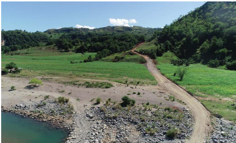
Construction of Access Road 2
