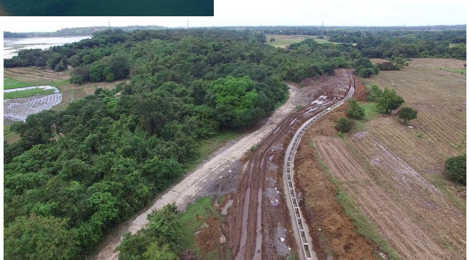
Construction of Canal Lining
