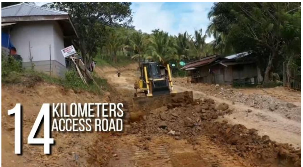
Construction of Access Road
