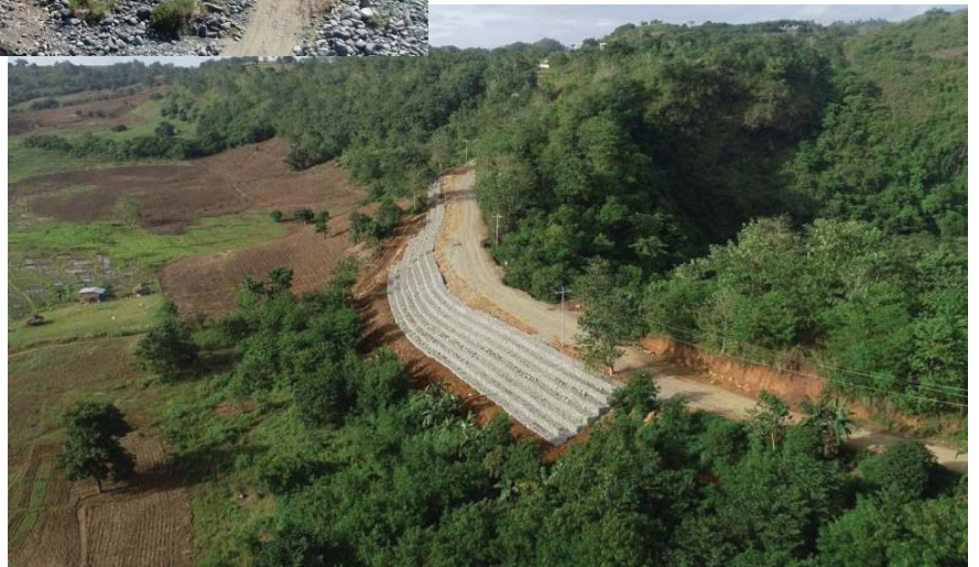
Construction of Sope Protection
