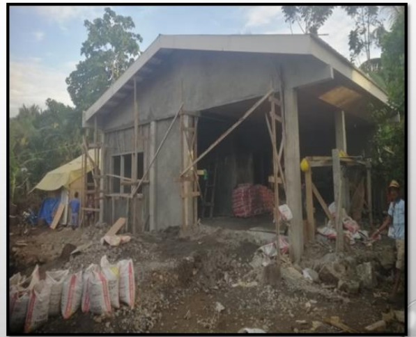
Construction of Project Facility
