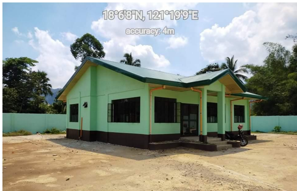
Completed LARIP Office
