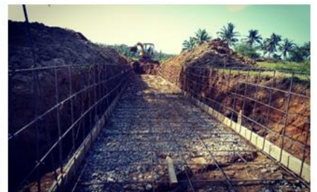
ON-GOING CONST. OF MAIN CANAL
