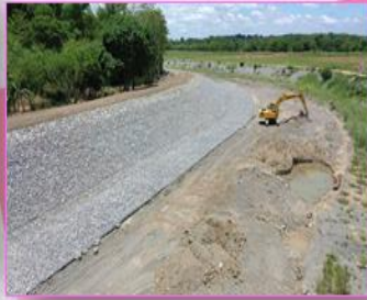
CONSTRUCTION OF SLOPE PROTECTION (STA. 25+295- STA. 25+868) OF BANILLA RIVER
