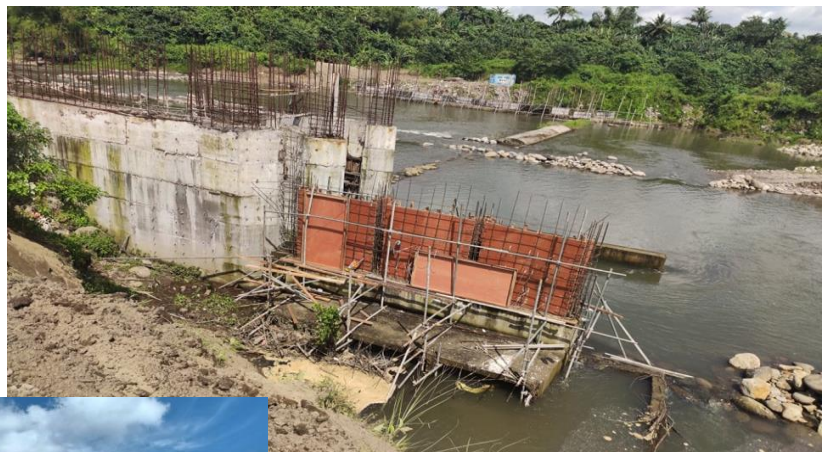
Ongoing construction of Diversion Dam
