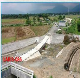
CONSTRUCTION OF OVERFLOW STRUCTURE (STA. 21+902) @ ADRI'S MAIN CANAL
