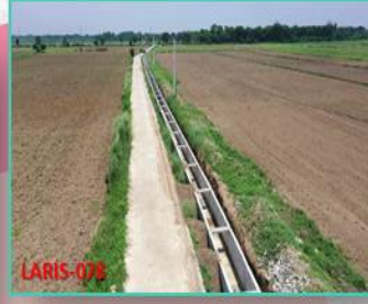
CONSTRUCTION OF RECTANGULAR CONCRETE CANAL LINING & APPURTENANT STRUCTURES (STA. 0+000-STA. 2+426.15) OF LARIS SUB-LATERAL B-1
