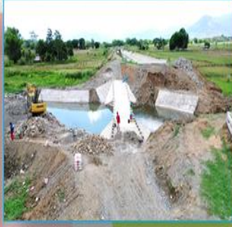
CONSTRUCTION OF OVERFLOW STRUCTURE (STA. 21+902) @ ADRI'S MAIN CANAL
