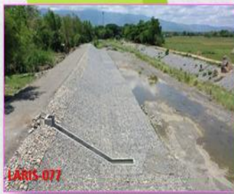
CONSTRUCTION OF SLOPE PROTECTION (STA. 25+295- STA. 25+868) OF BANILLA RIVER
