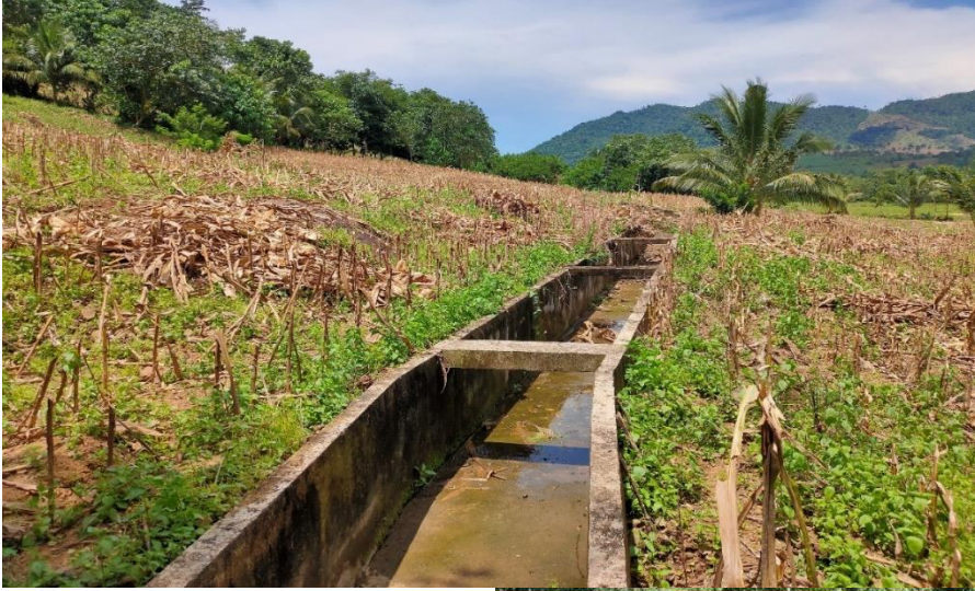
Canal Lining & Structures, BAYUYAN SRIP
