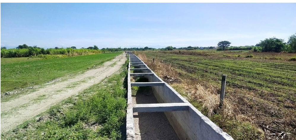
Construction of Lateral N
