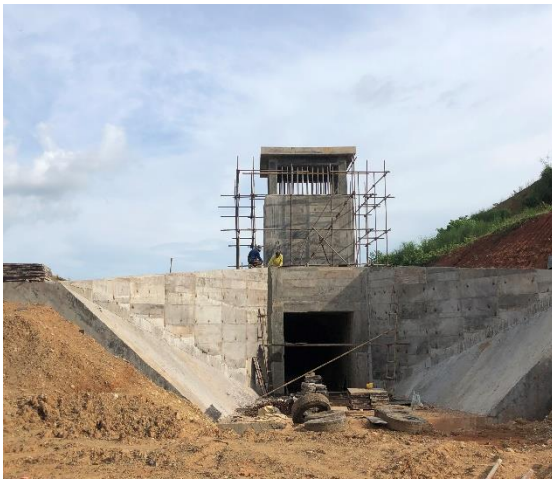
Construction of Embankment Dam, BALBALUNGAO SRIP
