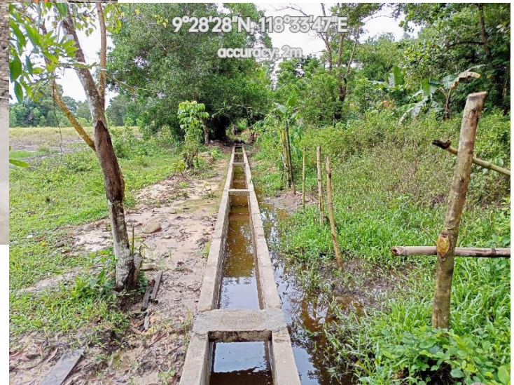
Construction of Spillway, IBATO-IRAAN SRIP
