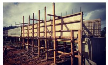
ON-GOING CONSTRUCTION OF ELEVATED FLUME MAIN CANAL @ STA. 15+955 TO 15+967
