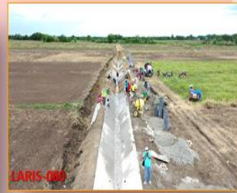
CONSTRUCTION OF RECTANGULAR CONCRETE CANAL LINING & APPURTENANT STRUCTURES (STA. 0+000-STA. 2+426.15) OF LARIS SUB-LATERAL B-1
