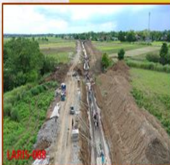
CONSTRUCTION OF closed conduit & appurtenant Structures (sta. 0+640 - STA. 1+184) OF LAGASIT SUPPLY CANAL
