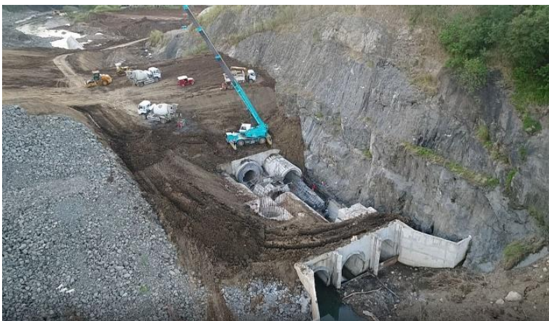
Ongoing construction of Diversion Conduit, BULO SRIP
