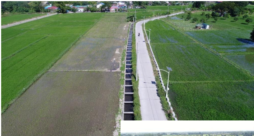
Construction of Canal and structures
