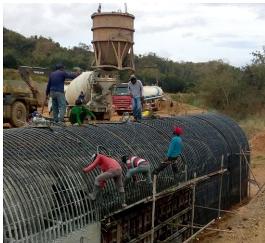
Concreting Works @ Diversion Conduit, Balbalungao SRIP
