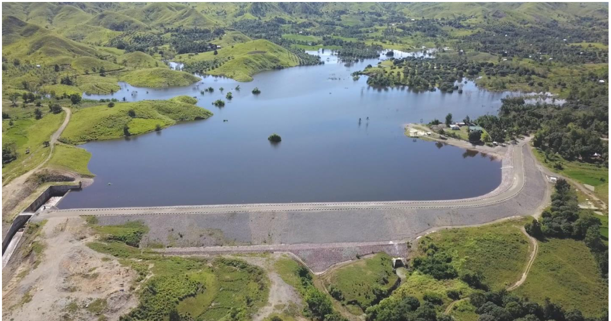
Completed Embankment Dam, BENLIW SRIP
