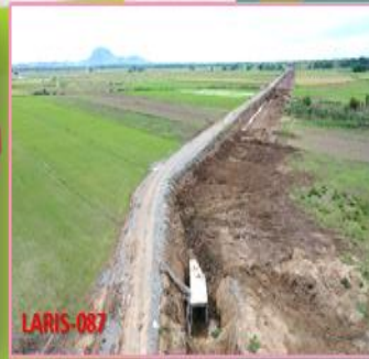
CONSTRUCTION OF closed conduit & appurtenant Structures (sta. 0+117) - STA. 0+640) OF LAGASIT SUPPLY CANAL
