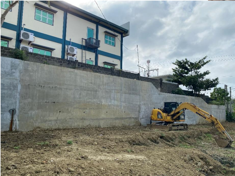
Office Building Slope Protection
