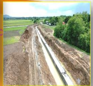
CONSTRUCTION OF CLOSED CONDUIT & APPURTENANT STRUCTURES (STA. 1+184-STA. 1+740) OF LAGASIT SUPPLY CANAL
