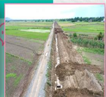
CONSTRUCTION OF closed conduit & appurtenant Structures (sta. 0+117) - STA. 0+640) OF LAGASIT SUPPLY CANAL
