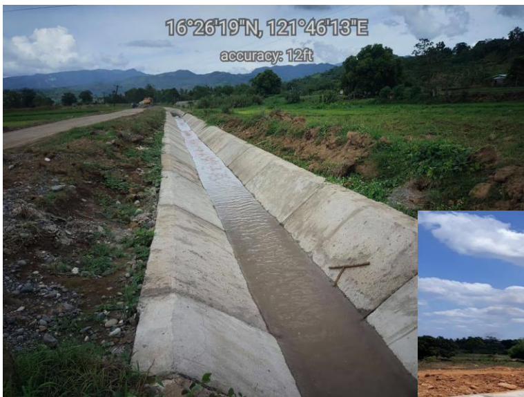
Construction of Irrigation Facilities
