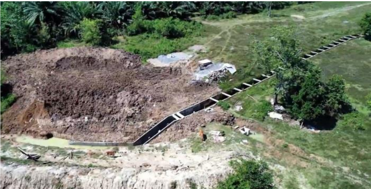
Completed Irrigation Facilities, TULUNAN SRIP
