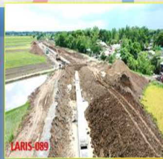
CONSTRUCTION OF CLOSED CONDUIT & APPURTENANT STRUCTURES (STA. 1+184-STA. 1+740) OF LAGASIT SUPPLY CANAL
