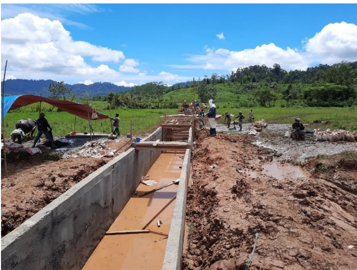
Construction of Main and Lateral Canals
