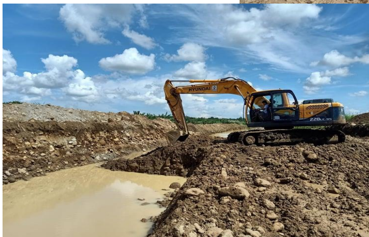
Ongoing construction of Main Canal
