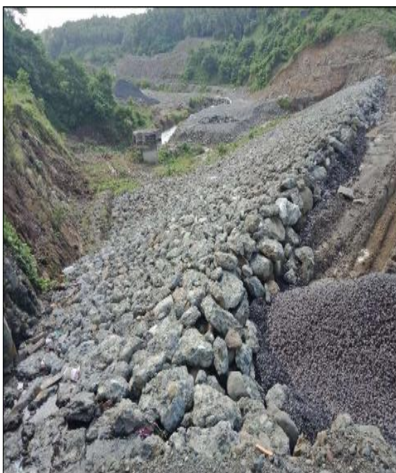
Gravel Bedding & Riprap, Spillway Area IBINGAN SRIP
