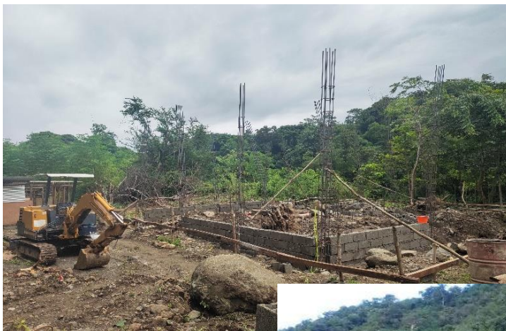
Completed Field Office, GACO SRIP
