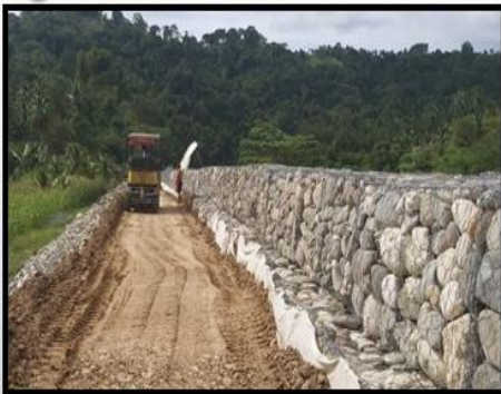
COMPLETED 245 METERS PROTECTION DIKE (PACKAGE 1)
