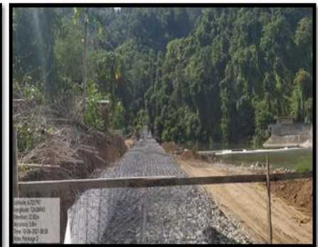
MECHANIZED EXCAVATION, INSTALLATION OF MATTRESS BOX, GABION BOX AND FILTER CLOTH (PACKAGE 2)
