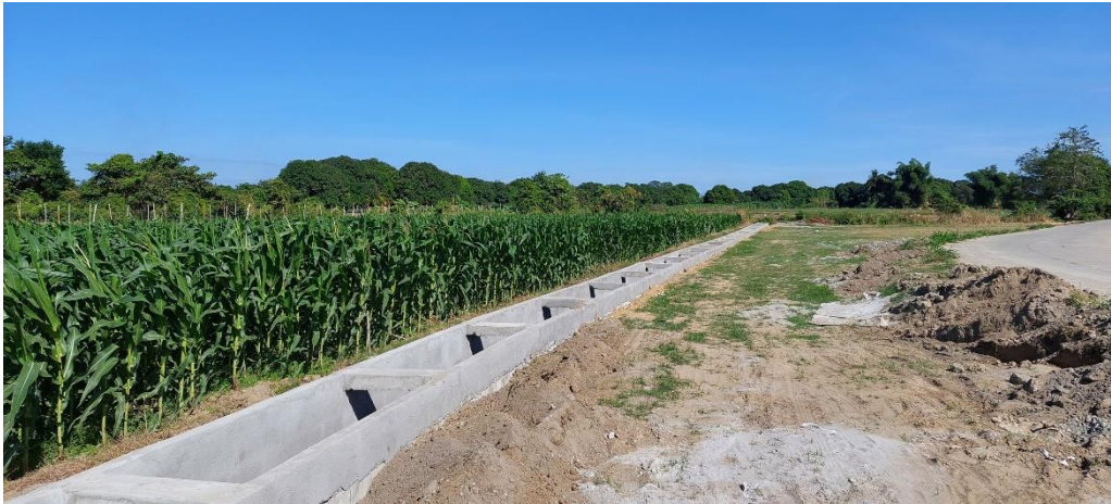
Construction of Lateral C-1
