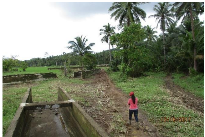
MAIN CANAL TYPHOON DAMAGE (STA 3+380 – 3+540, 3+720 – 4+140)
