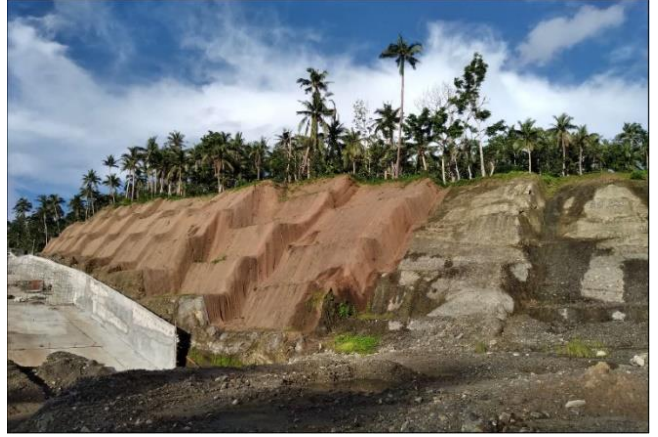
SPILLWAY COCO FIBER NET
