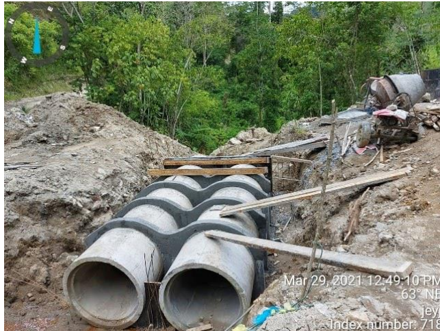
INSTALLED RC PIPES WITH COLLAR AT STA. 5+755
