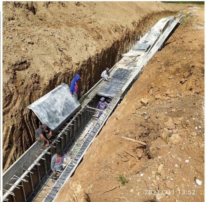
Ongoing Concreting works of Closed Conduit at Station 7+260 - 7+560
