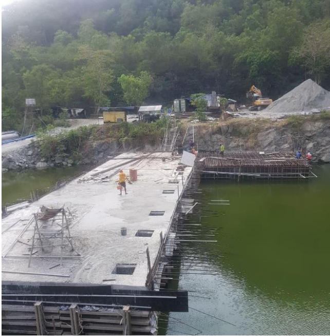
Completed top slab of Sump Intake
