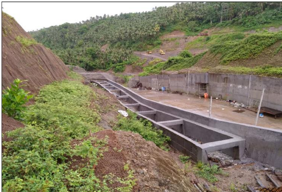
COLLECTOR CHANNEL AT SPILLWAY AREA LEFT SIDE FACING DOWNSTREAM
