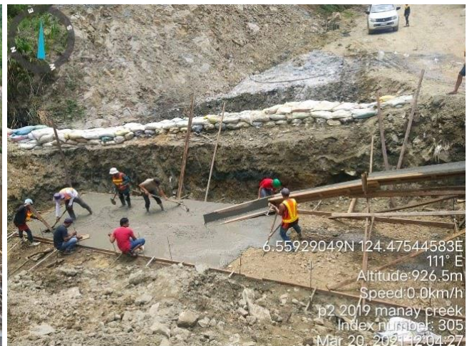
ONGOING LEAN CONCRETING ON MANAY CREEK STRUCTURE
