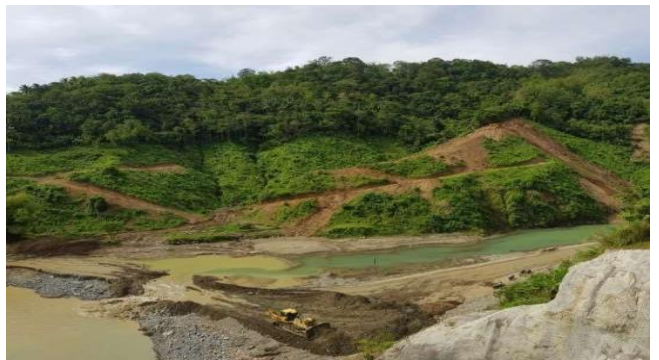
CLEARING AND EXCAVATION FOR AFTERBAY DAM BODY RIGHT BANK SLOPE BENCHING AT EL.150-160
