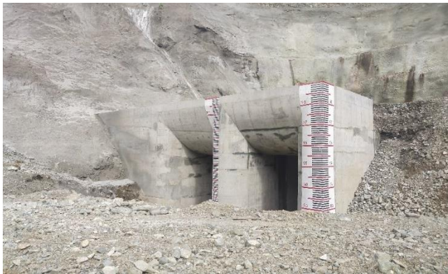
COMPLETED DIVERSION TUNNEL (INLET)
