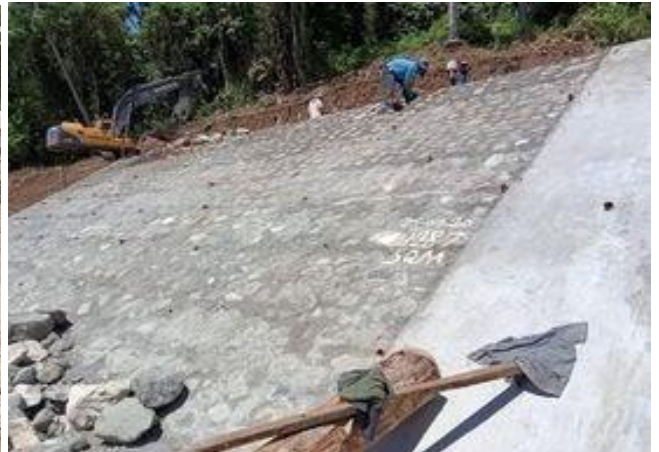
ON-GOING CONSTRUCTION OF INCLINED WALL
