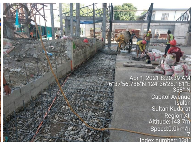
DURING POURING OF CONCRETE ON SLAB
