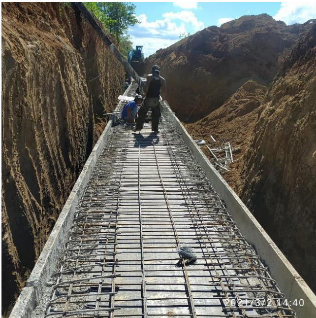
Ongoing Concreting works of Closed Conduit at Station 7+260 - 7+560
