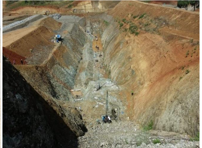
DRILLING AND GROUTING AT DAM CORE TRENCH
