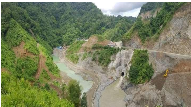
CLEARING AND MAKING OF ACCESS FOR AFTERBAY DAM BODY RIGHT BANK SLOPE
