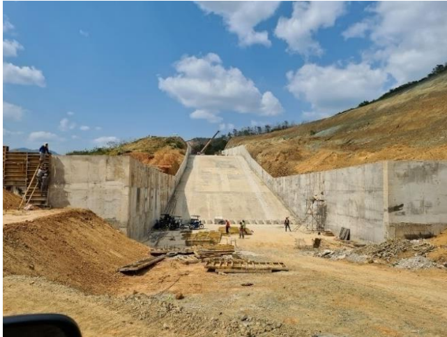
CONCRETING WORKS AT SPILLWAY STRUCTURE
