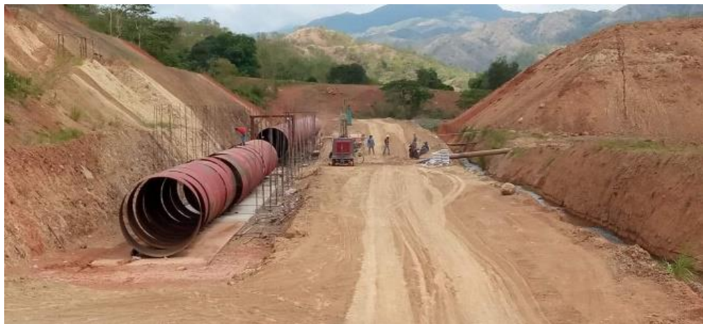
FABRICATION AND INSTALLATION OF CONDUIT PIPES
