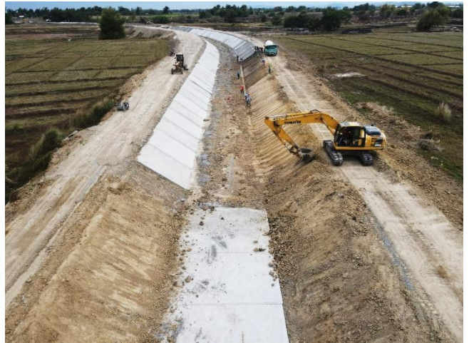
Ongoing construction of canal lining at South Main Canal Package 2, from Sta. 11+400.00 to Sta. 11+500.00
