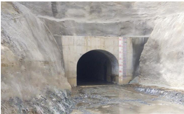
COMPLETED DIVERSION TUNNEL (OUTLET)
