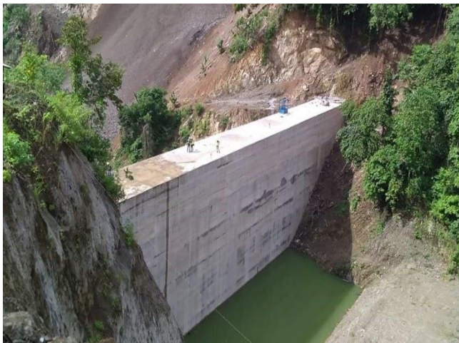
COMPLETED COFFER DAM (UPSTREAM)
