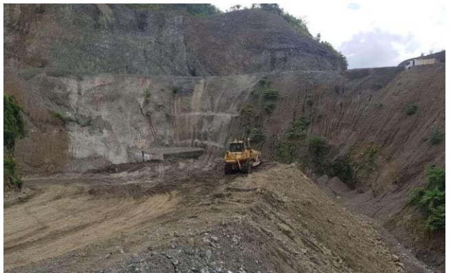
SPREADING OF AGGREGATES NEAR FABRICATION AREA D/S OF INLET OF AFTERBAY AREA.
