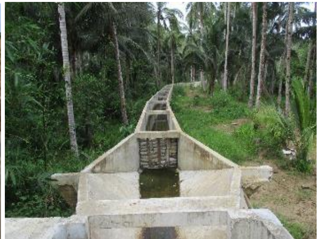
MAIN CANAL – ELEVATED FLUME & SIPHON #3 (STA. 5+561-5+744)
