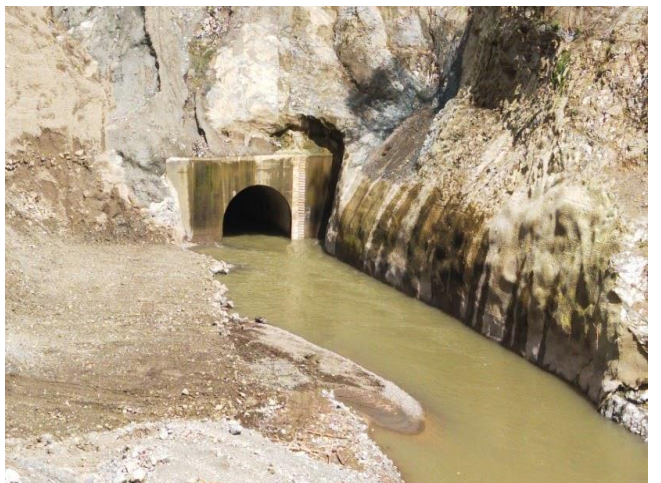
COMPLETED DIVERSION TUNNEL (OUTLET)
