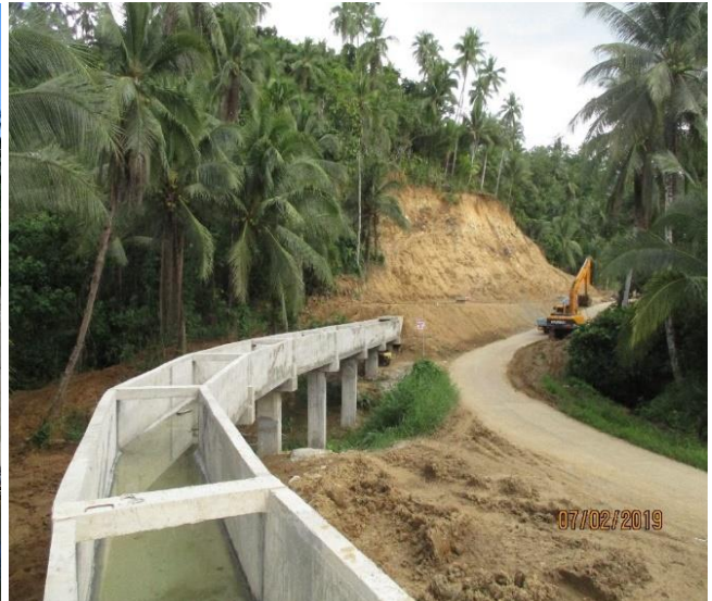
MC- ELEVATED FLUME & CUT & COVER INCLUDING ROAD CROSSING (STA. 6+940-7+105)
