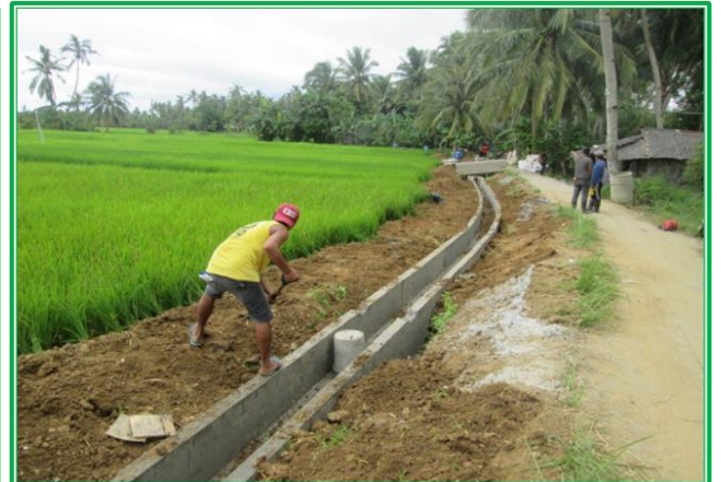
BACKFILLING WORKS AT MFD A-15 ALONG LATERAL A
