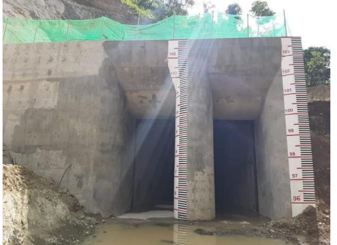
COMPLETED DIVERSION TUNNEL (INLET)
