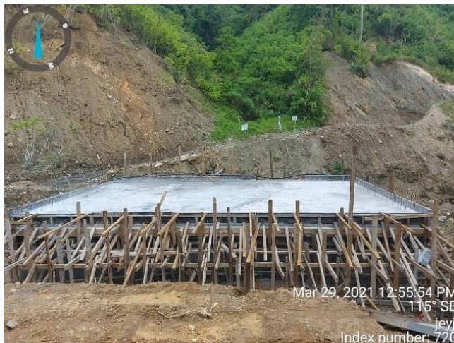
FALSE WORK AND CONCRETE TOP SLAB OF SALATAN STRUCTURE
