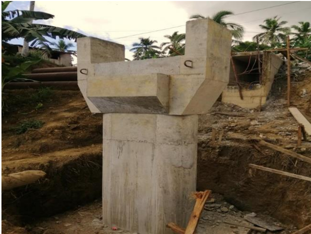
BRIDGE FLUME ALONG LATERAL A
