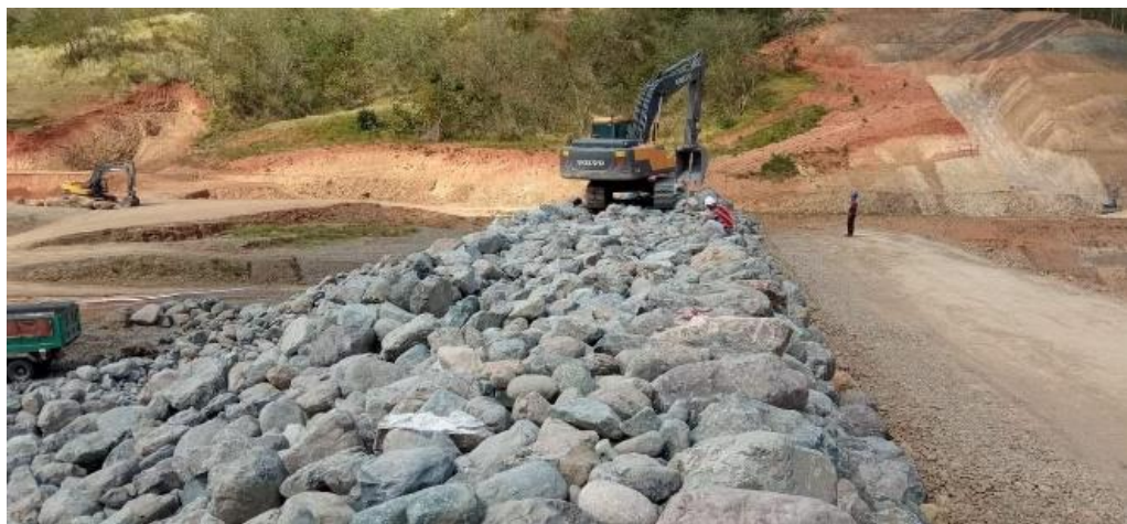
CONSTRUCTION OF ROCK TOE
