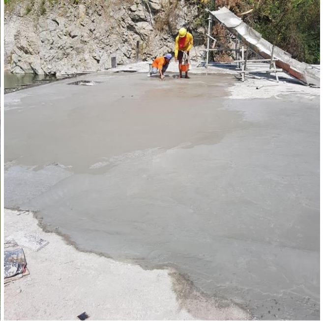
Completed top slab of Sump Intake
