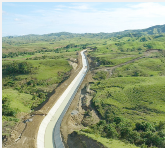
Construction of Main and Diversion Canal of CRPIP in Pinukpuk, Kalinga
