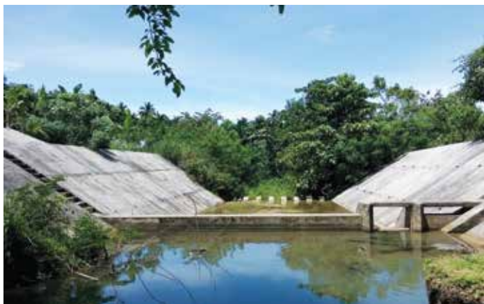
San Roque Communal Irrigation System San Roque, Pilar, Surigao Del Norte
