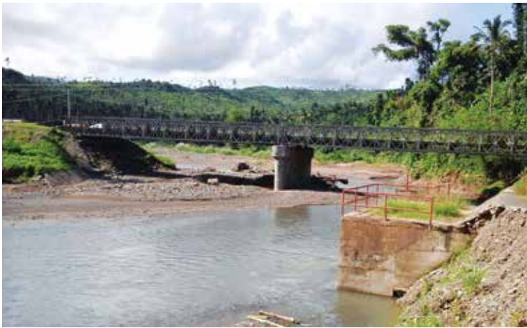
Baclinan Communal Irrigation System Boston, Davao Oriental
