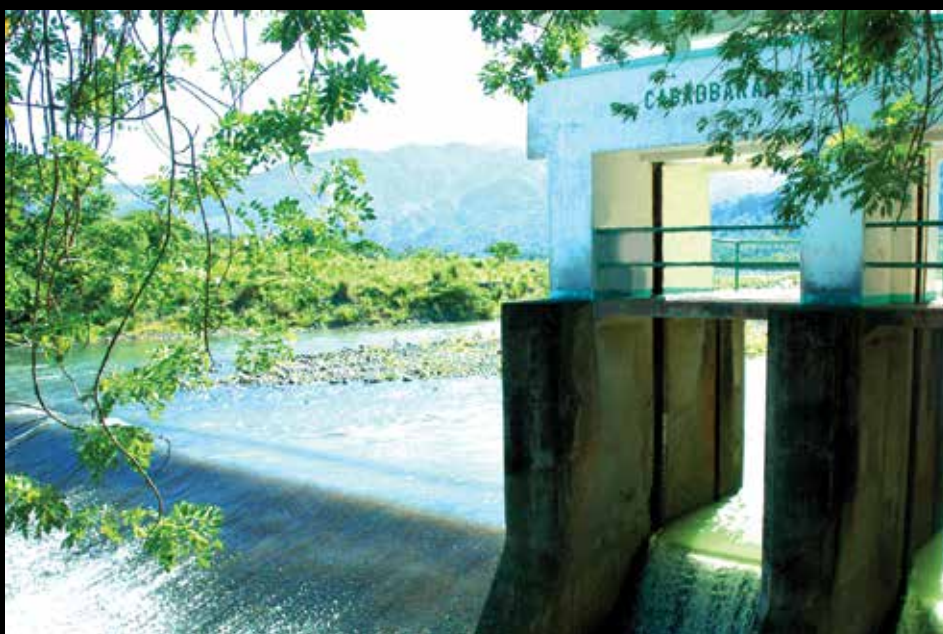
Cabadbaran Dam Calamba, Cabadbaran City
