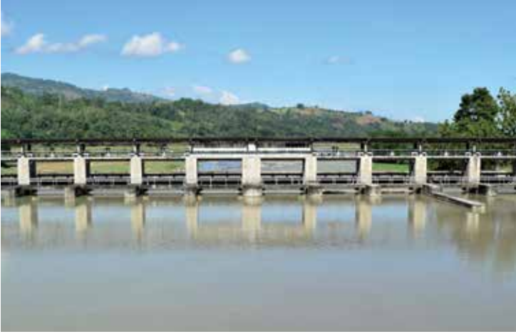
Allah River Irrigation System Surallah, South Cotabato
