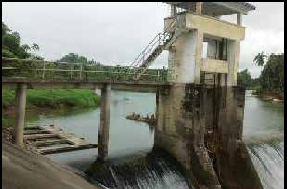
Saug River Irrigation System Asuncion, Davao del Norte
