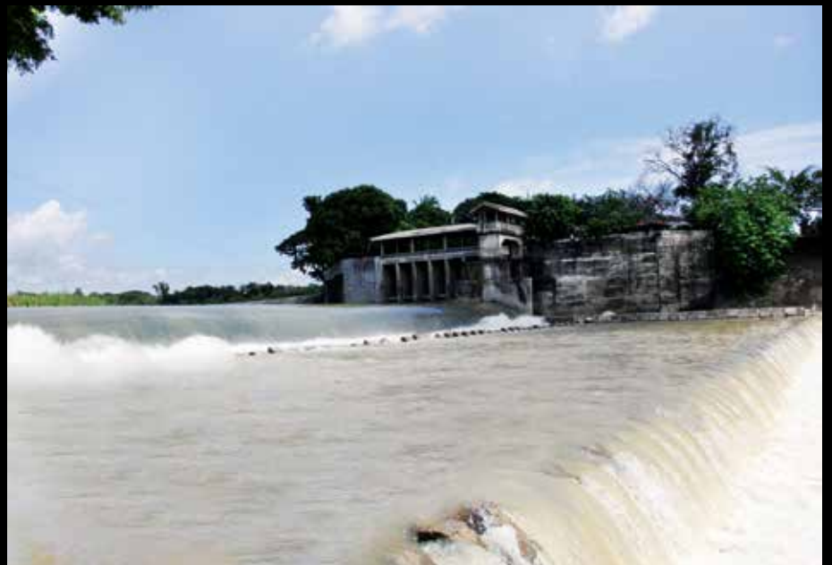
Sta. Barbara River Irrigation System
