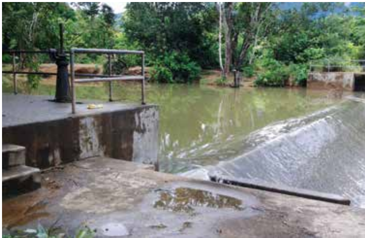
Tampayan Communal Irrigation System Tampayan, Magdiwang, Romblon
