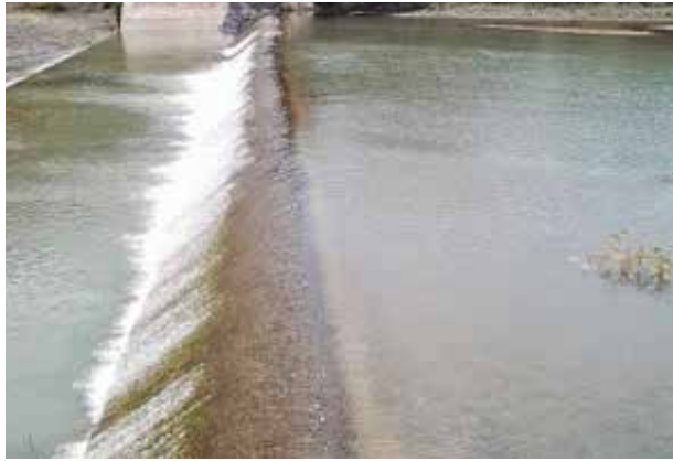
Bugasong Communal Irrigation System Bugasong, Antique
