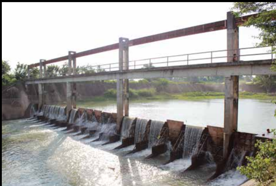
Mangindong Dam Brgy Luacan, Dinalupihan, Bataan
