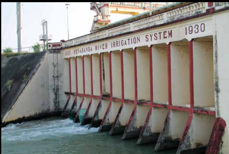
Penris Dam (Division 4) Gapan City, Nueva Ecija.
