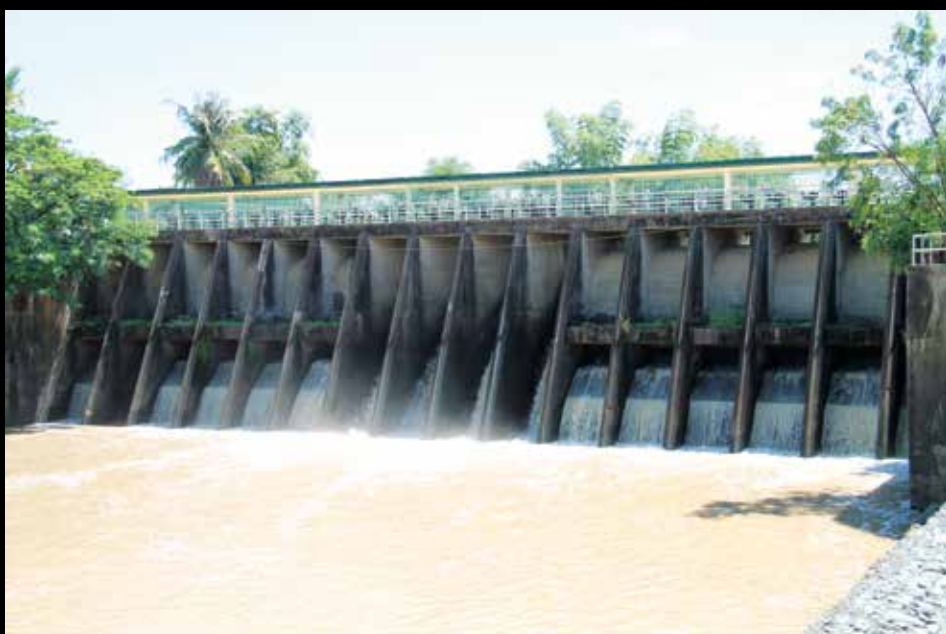
Murcon Dam (Division 2) Nueva Ecija
