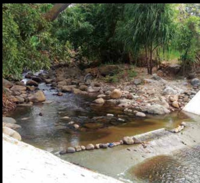
Banayam Dam Bagak, Bataan
