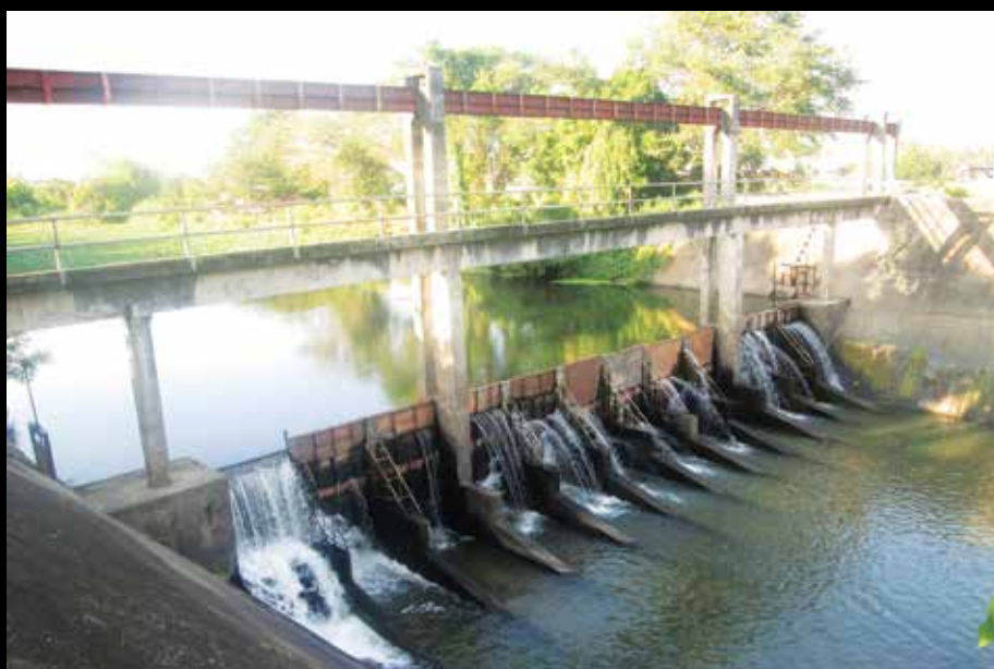
Layac Dam Dinalupihan, Bataan
