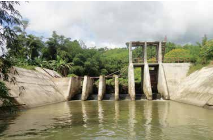
Baluran-Tipil Irrigation System Tungawan, Zamboanga Sibugay
