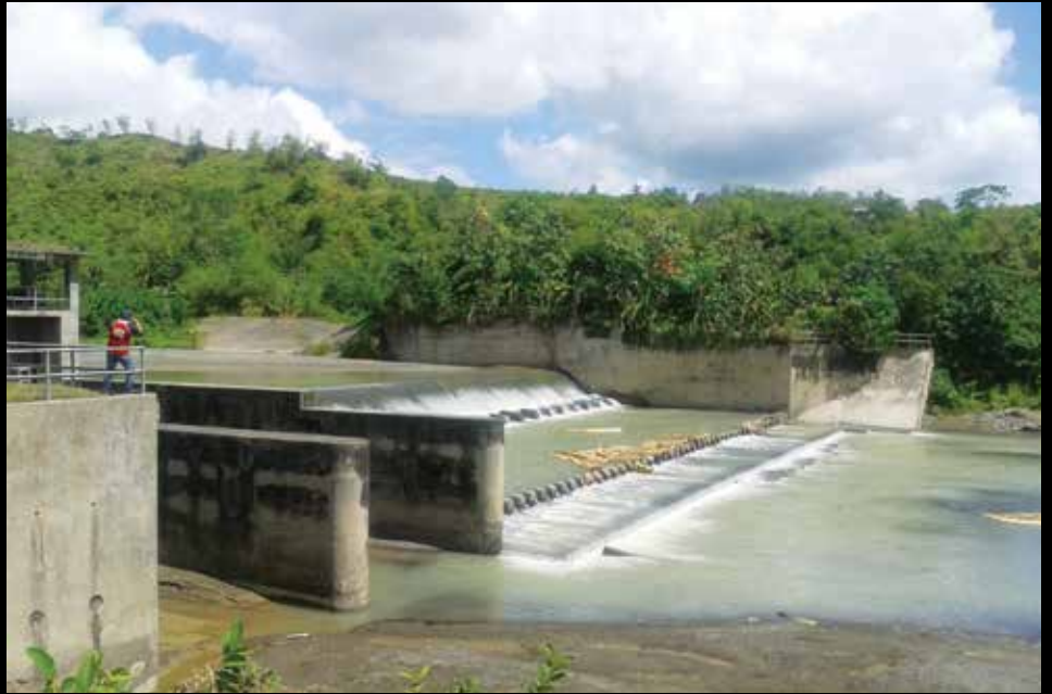
Kipaliku River Irrigation Suystem Sto. Tomas, Davao del Norte
