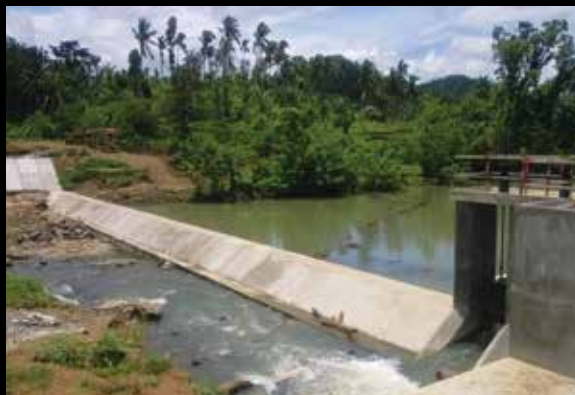
Agbalili Communal Irrigation System
