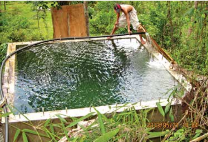
Ambingel Communal Irrigation System Tuba, Benguet
