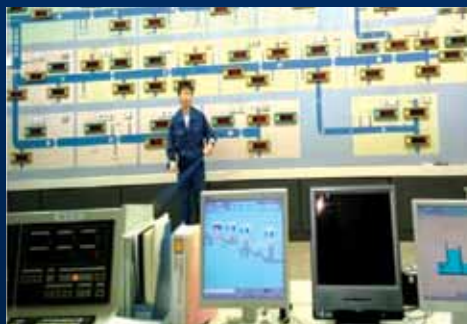
Control Room of Miyata Irrigation System -Monitoring of the status of irrigation water flows in each facility within the irrigation system.
