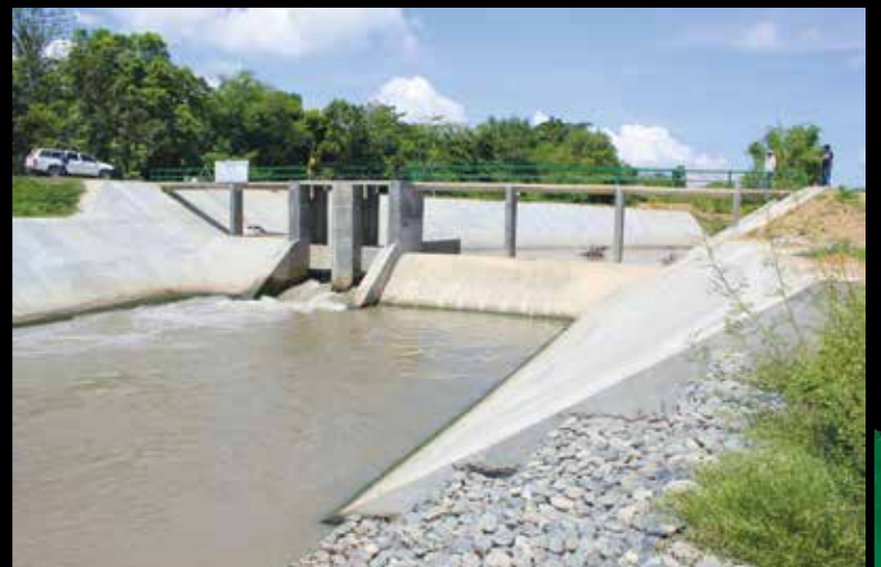
The Patanad Diversion Dam is a drainage reuse structure in San Isidro, Isabela. It is expected to irrigate 200 hectares of farmlands currently planted to corn.
