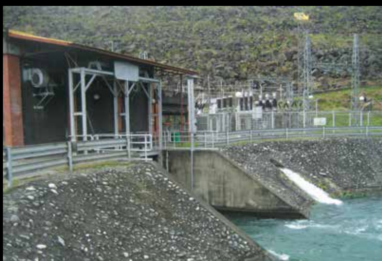
The Baligatan Diversion Dam delivers water to the South High Canal and Oscariz Canal serving the high level areas in the system.
