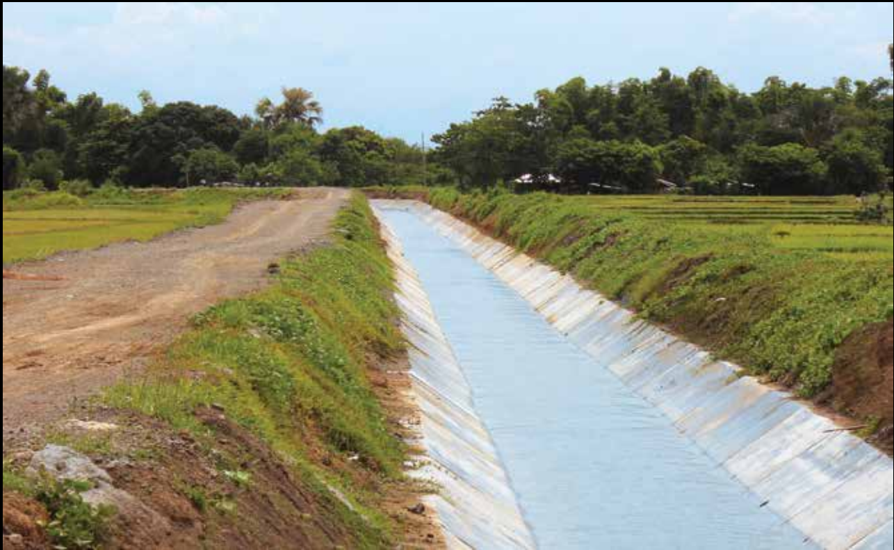
Concrete-lined lateral
