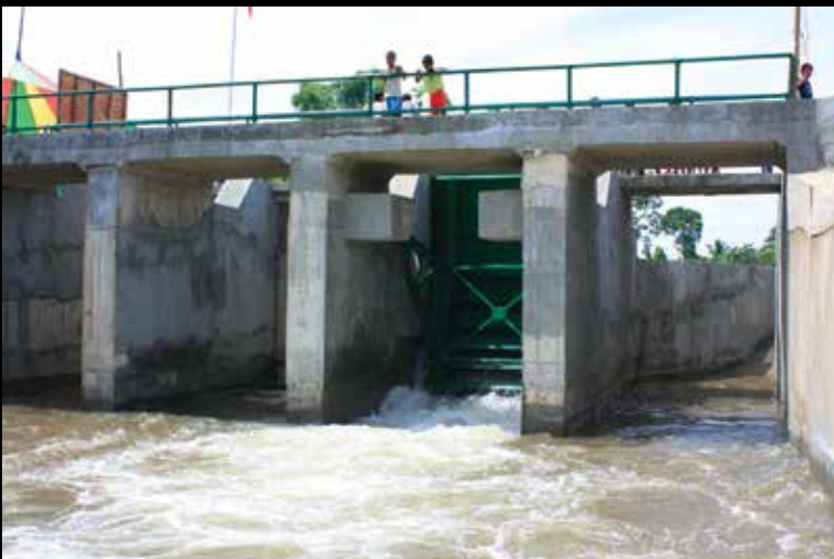
The Balaobao Checkgate No. 3 along the Balaobao Creek in Cabatuan, Isabela is a drainage reuse structure which serves 1,000 hectares of ricelands. The checkgate was constructed in 2010.
