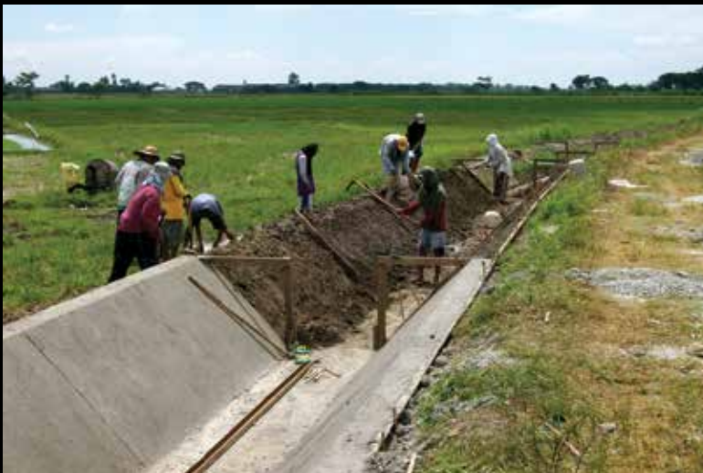
Concreting of Canal Lining at Lateral B-3, TARRIS Area, Brgy. Guevarra, La Paz, Tarlac
