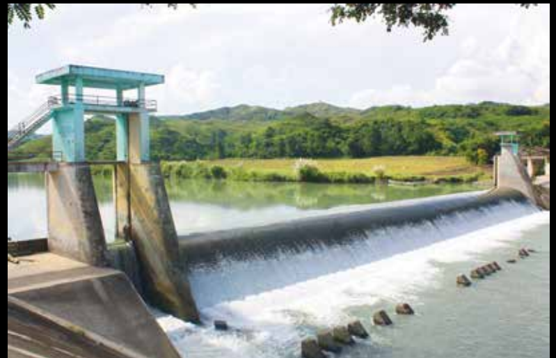
The Siffu Dam is a run-off-the-river type dam serving 5,905 hectares of ricelands in the municipalities of Roxas, San Manuel and Quirino in the province of Isabela.
